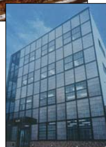
PV Integrated in Office Glazing Photo Credit: Solar Design Associates (IEA PVPS)
